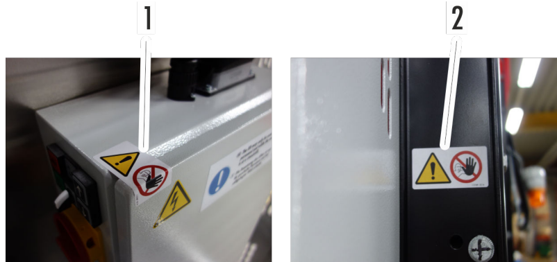
Fig. 6: Seal on control cabinet and overload
