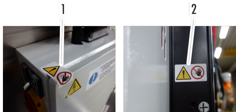
Fig. 8: Seal on control cabinet and overload
